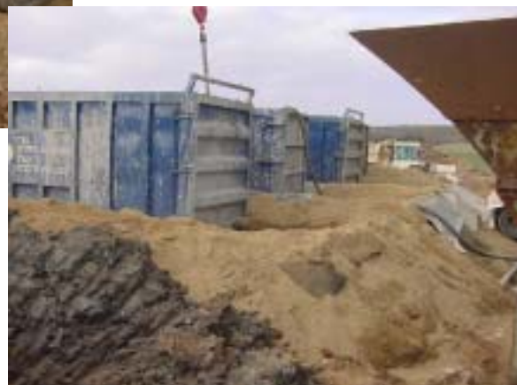
The large storage containers on site for the oily drilling waste
